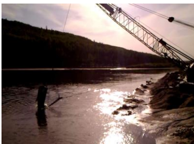
October – Cleaning Up The Snye
