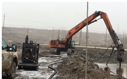
Long Reach Excavators
