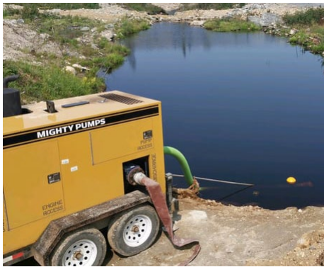
Water Management Plan in Action with a Dewatering Pump
